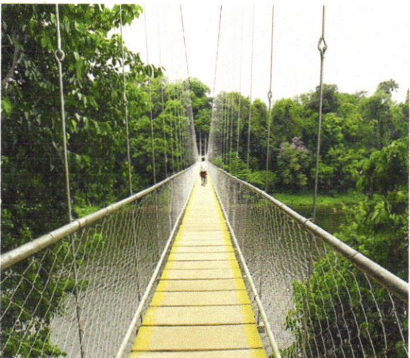
Bridge over Chaliyar river
